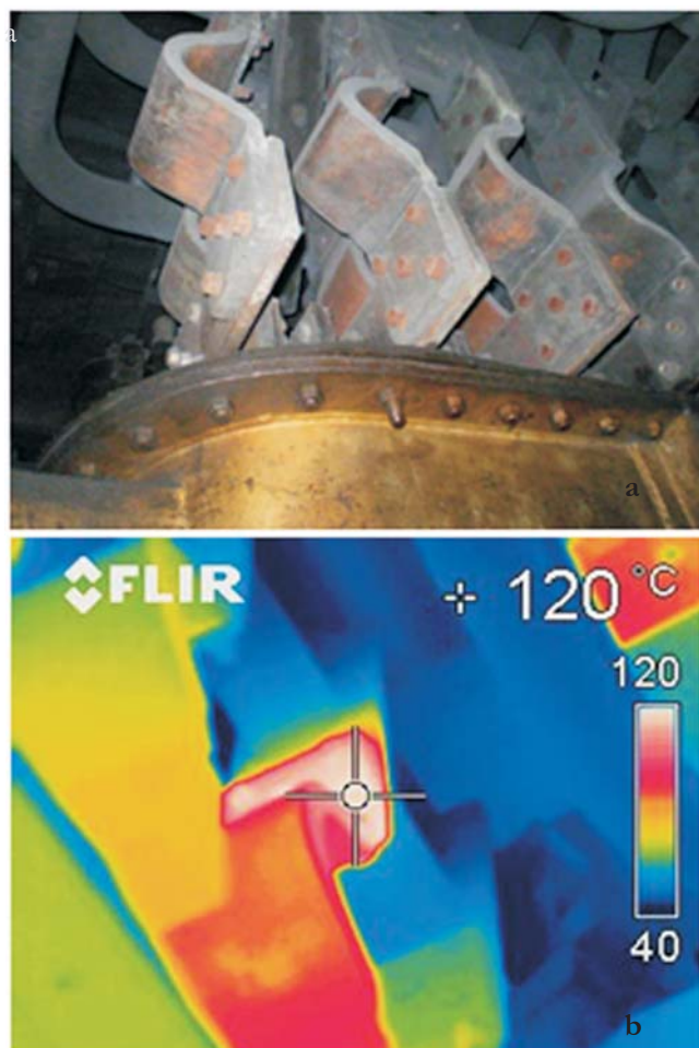
Figure 1 Electric connections of bus-bars supplying the arc furnaces: a) bus-bars, b) thermograms
